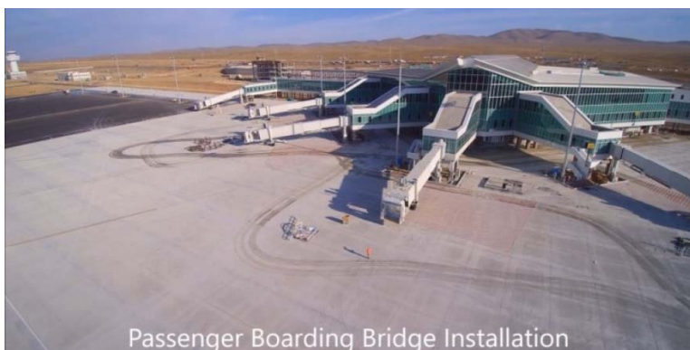
Photo2 NUBIA Construction Project (Mongolia) as of .May 17 th . 2016
